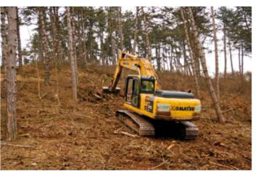
Clearing of tree crown cuttings and uprooting of rootstocks using an excavator
